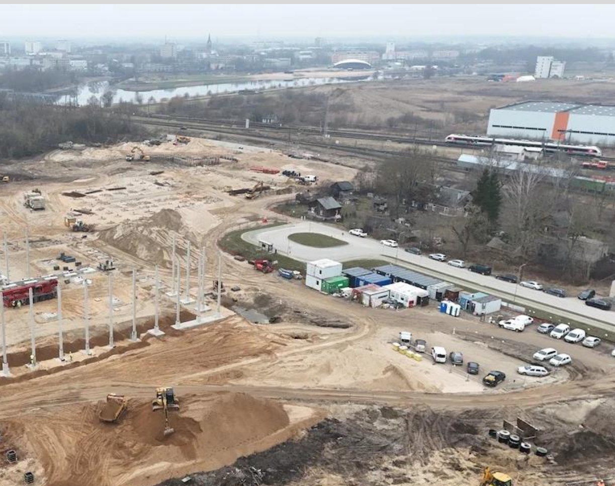
Construction of pea protein and starch production plant
